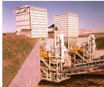
Black Thunder, Wyoming; Semi-Mobile Truck Dump and Crushing Stations
